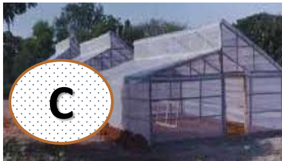
Greenhouse with Oakwood structure covered with an LDPE-based plastic film (Greenhouse “C”).
