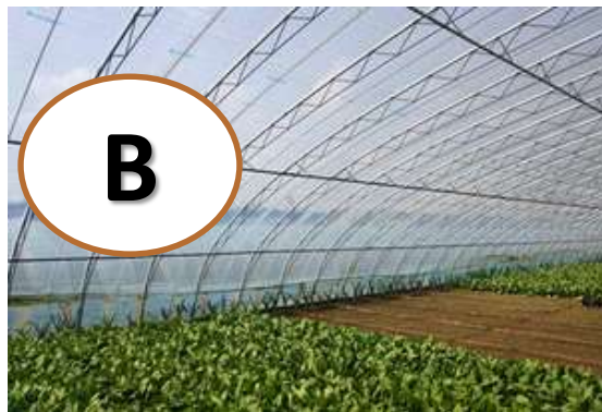
Tunnel shaped zinc-coated steel structure covered with an LDPE-based plastic film (Greenhouse “B”).
